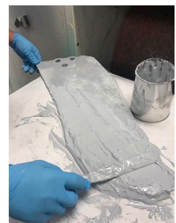
2. Corroded edges of mixing blades being replaced with metal mesh and filled in with Novocoat EP3300 Paste/Caulk.
